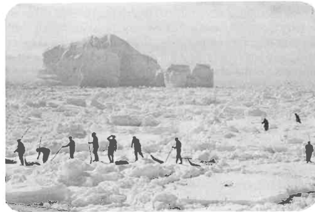
FIG. 80. (Upper) Shades of former glory. M/V Arctic Prowler leaves St. John's for the icefields, March 6, 1953. This type of sealer was an ex World War II boom defence vessel; (Lower) Men from Algerine "double-panning" (making larger piles of pelts) in tight ice, March 13, 1953. Note the gaffs, then used to kill seals.
